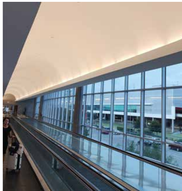
Fluorescent Bulbs create gaps in lighting
